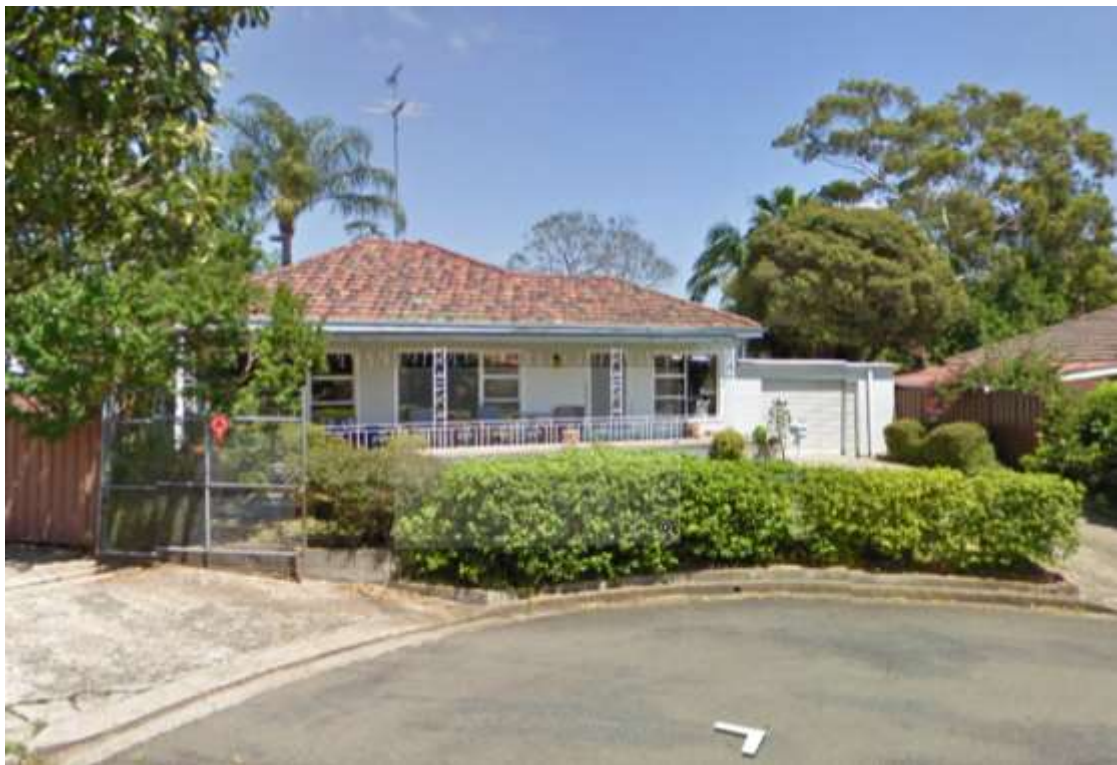
8 Hannah Street to be demolished
