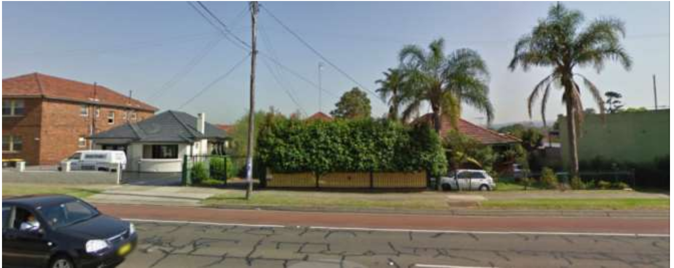
View from Great Western Highway of existing dwellings to the west
